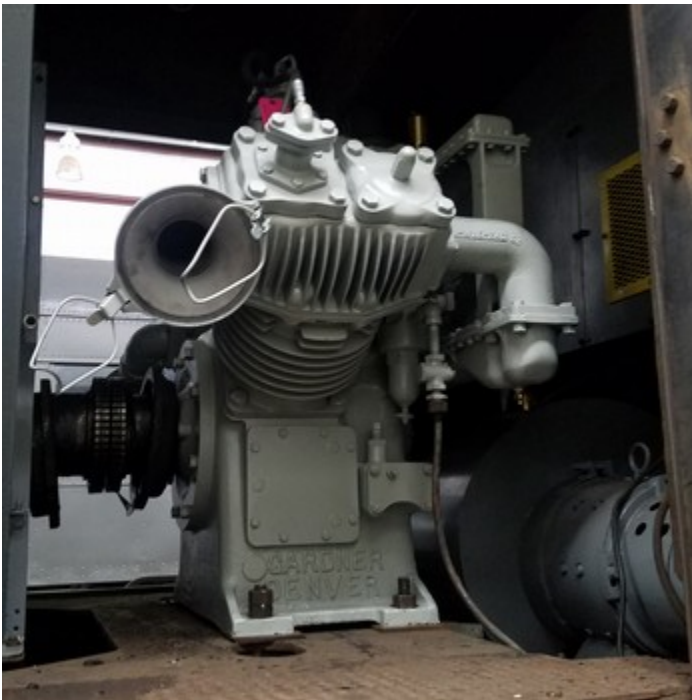
Engine No 709's compressor installed. John Sprinkle
