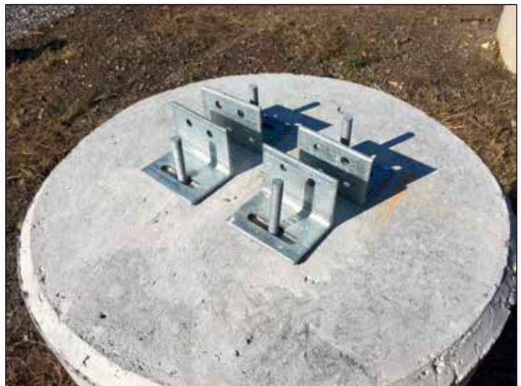
All: Lewis Foster Photos Top: Completed painting on the mule. Middle: N&W 512's completed window frames. Bottom: poured concrete base and brackets for structure.
