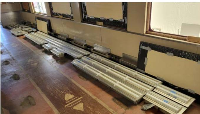
generator. The fixtures will also be cleaned and polished to remove 70 years of tarnish and paint.
