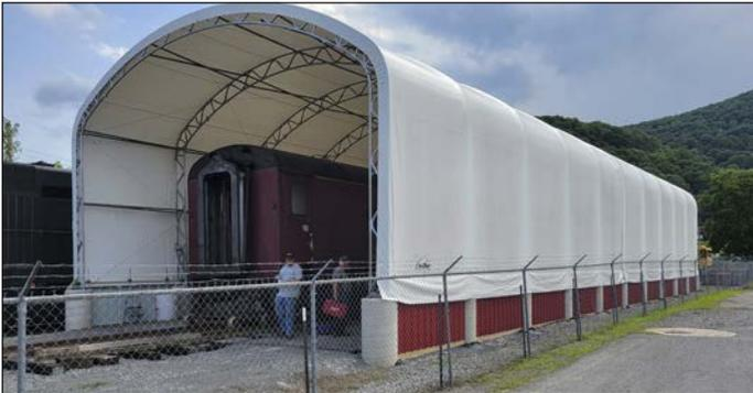
We've continued working on the car shelter over the summer as well. The sheet metal sides have been installed between the foundation columns along both sides of the building and the drainage on each side has been finished. A workstation with a back wall to protect the cloth of the building cover has been set up as well. Cloth covers to allow both ends of the building
