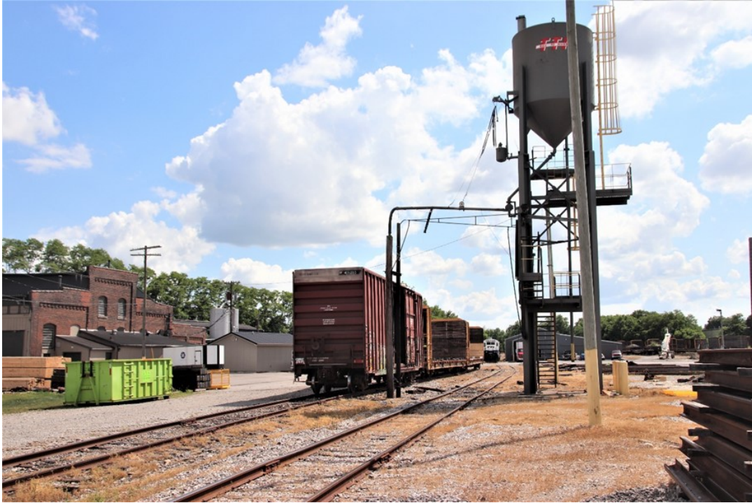
The Paris Yard sand tower still stands proudly bearing the "TTI" logo
