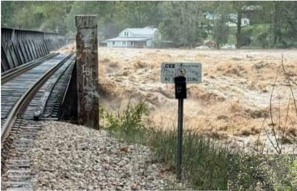
CSX bridge over Nolichucky River at Chestoa, TN.
