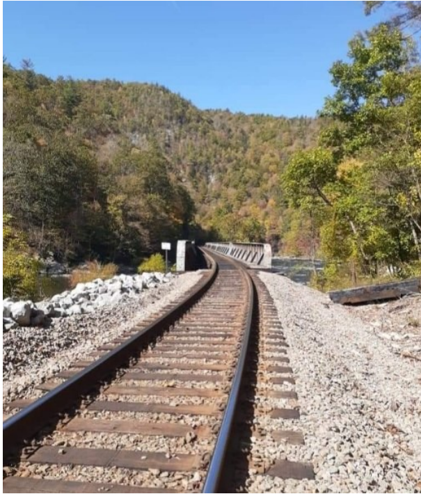
Top: CSX bridge at Poplar, NC before Helene.
