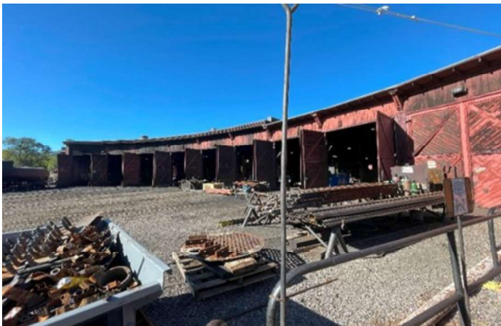
The outside of the working D&SNG roundhouse at Durango.
