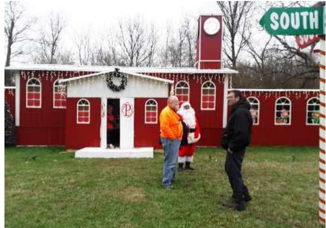
Front elevation of the castle. The taller part of the structure is built on a trailer. The clock tower is raised and lowered using a pulley system and cables. The lower walls extend the size of the castle on both sides. They are attached to the outside of the main castle for transportation.
