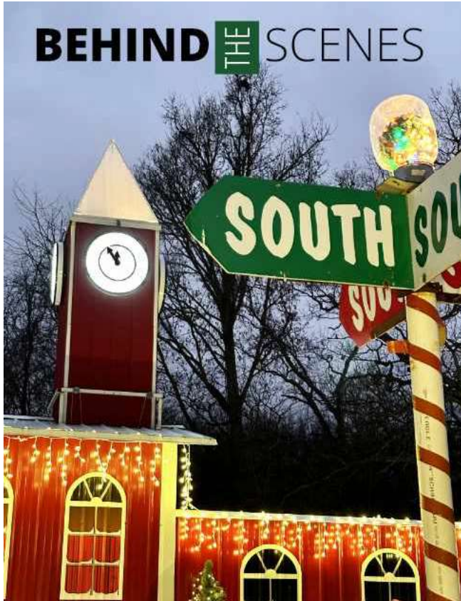
Front elevation of the castle. The taller part of the structure is built on a trailer. The clock tower is raised and lowered using a pulley system and cables. The lower walls extend the size of the castle on both sides. They are attached to the outside of the main castle for transportation.
