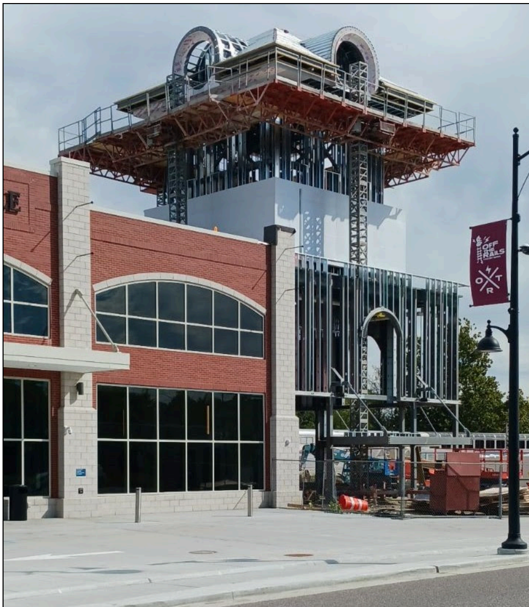
The distinctive tower was still under construction.
