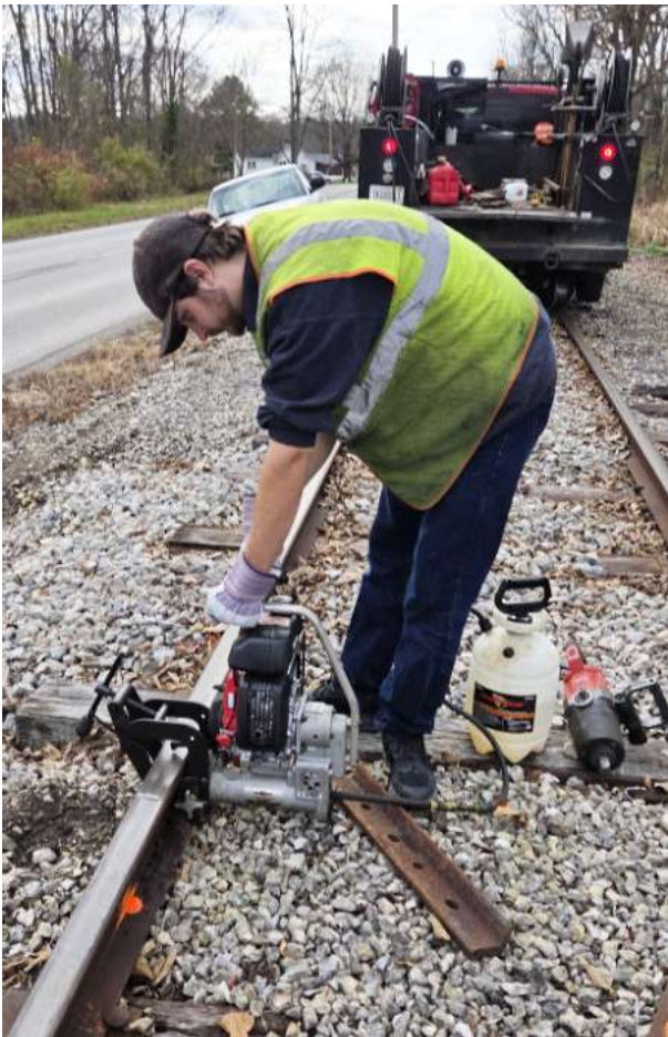
Nic McCoy, Steve McCann and Travis Weller responded to the broken rail on the Alpine straight. At this point the railroad is alongside Indiana Route 121. In this photo Nic is drilling holes in the rail prior to bolting on the joint bars. One of the bars is by Nic's left foot.
