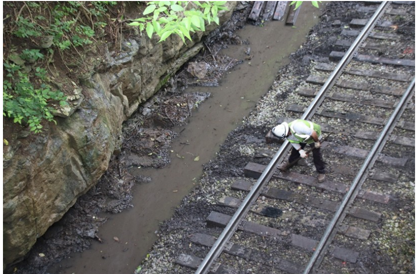
Pulling a misdriven spike
