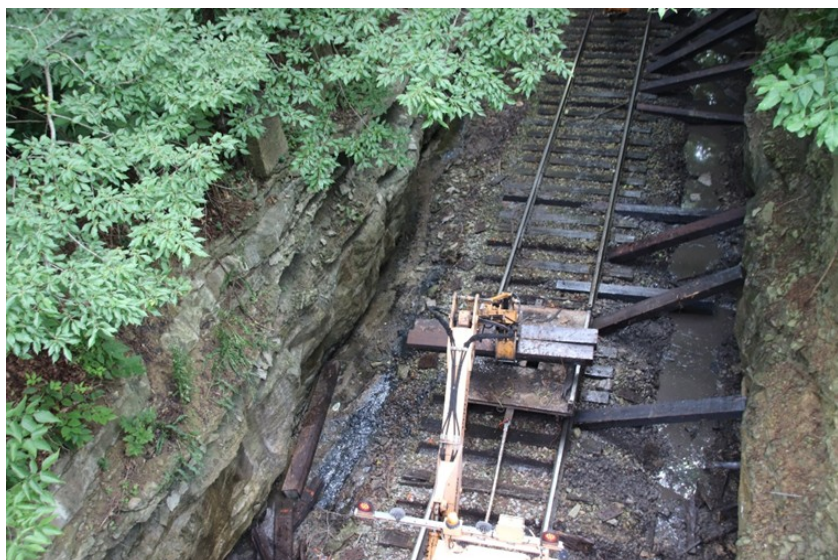
New ties stacked for insertion
