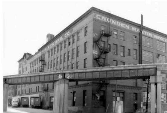
Rail line at Northeast corner
